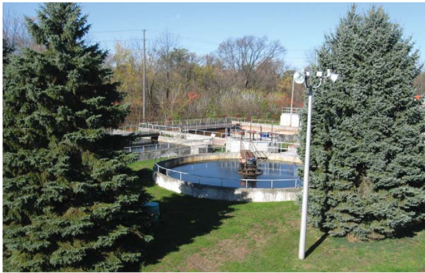
Plant two's secondary clarifiers.
