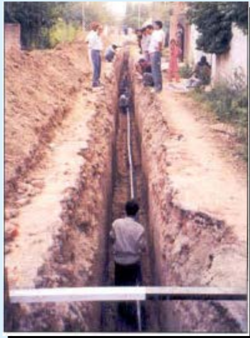
Siphon to flush upstream sewers
