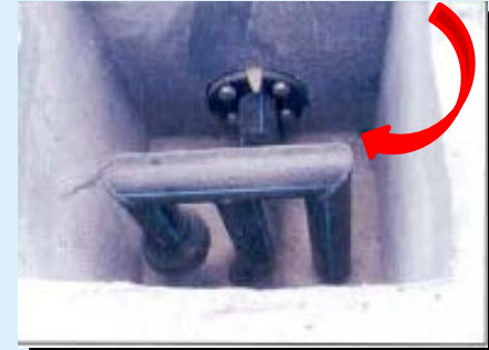
Siphon to flush upstream sewers
