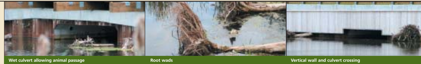
Wet culvert allowing animal passage
